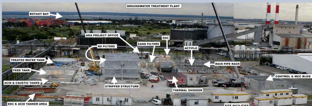
Plant layout during construction.
