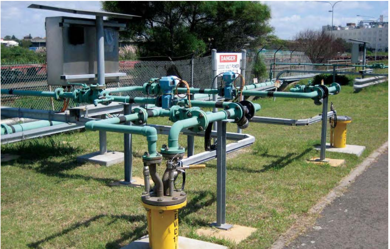
The extraction wells pump water from the shallow, intermediate and deep aquifers, thereby containing the contaminated groundwater within three areas.
