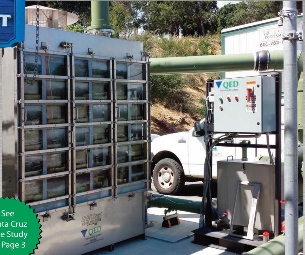
**The E-Z Tray® Air Stripper is a sliding tray, stainless steel air stripper used to remove volatile organic compounds (VOCs) from contaminated groundwater and waste streams. The exclusive design of the E-Z Tray stripper results in very high removal efficiencies in an easier-to-maintain process unit.**
