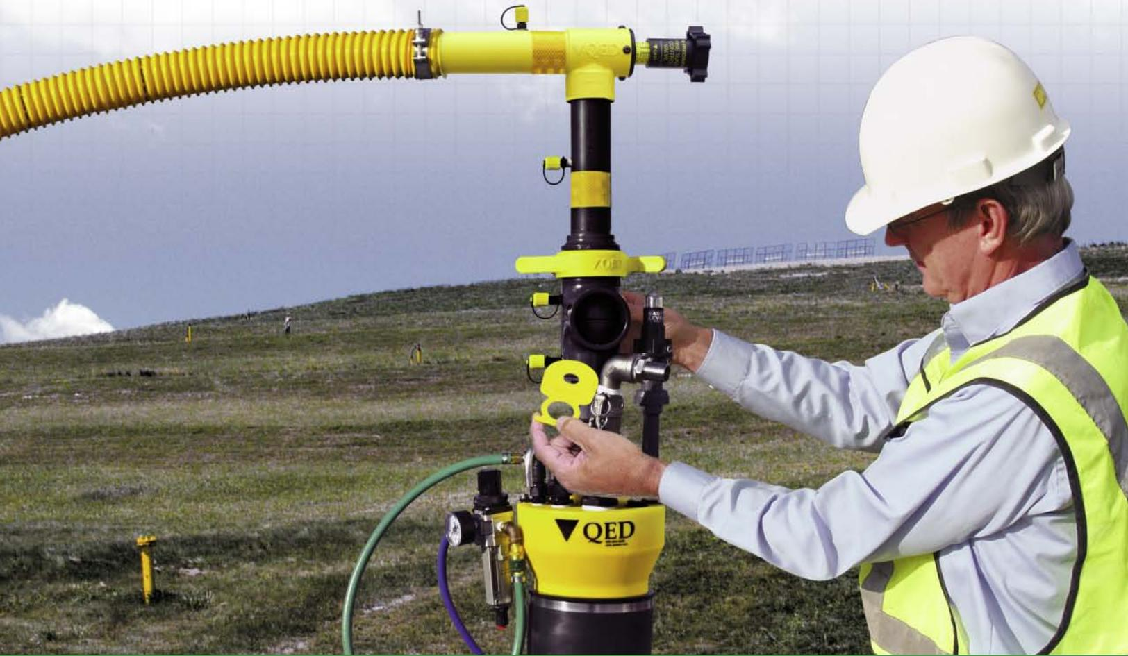
*New wellheads reduce balance gas and oxygen concentrations while increasing or maintaining a steady flow of methane.*
